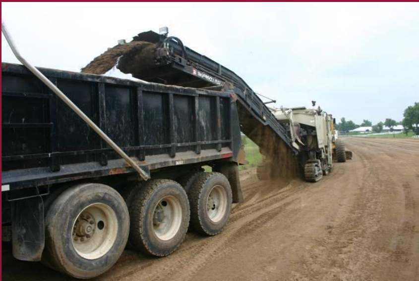
Removal of dirt surface
